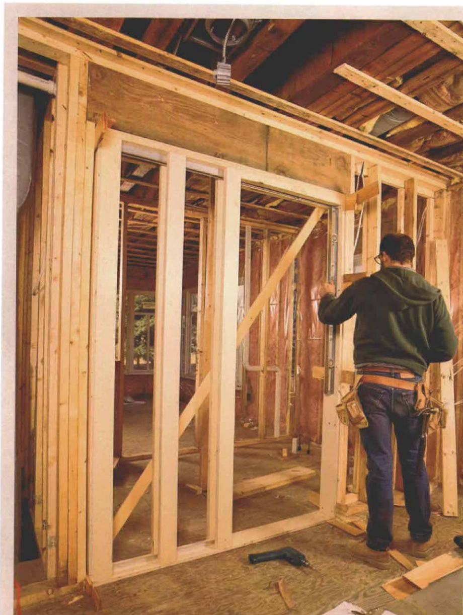
The Woodmeister Corp. builds pocket-door frames as a unit in the shop and ships them to the job site squared and braced. Above, Jeff Ham plumbs the strike-side of the pocket-door frame. The plywood plate running across the doorway will be cut out after the frame installation.
